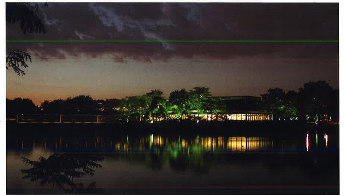
Site and landscape illumination were added to this attractive building to give it a stronger presence across the water in the evening darkness.
